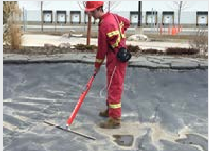
Figure 5. Arc Testing on an exposed geomembrane
