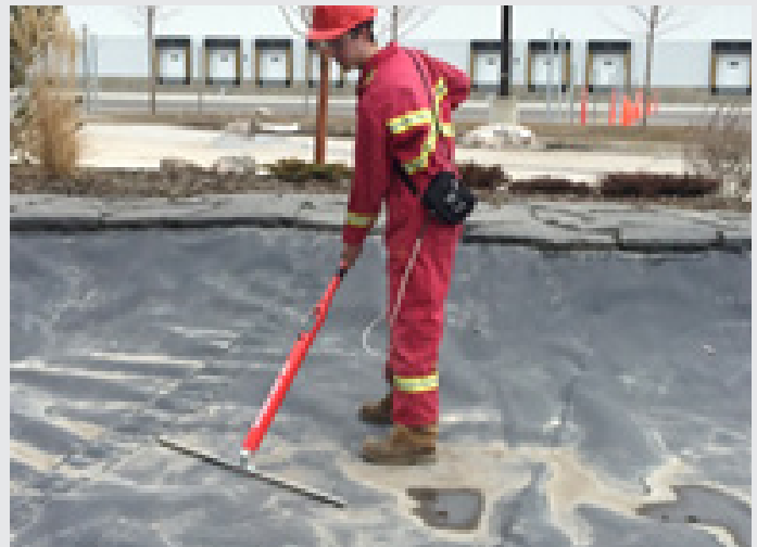
Figure 5. Arc Testing on an exposed geomembrane
