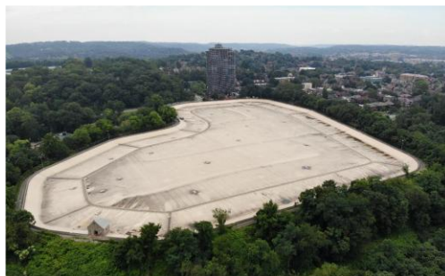
Figure 15. Aerial of Highland 2 Floating Cover in application.
