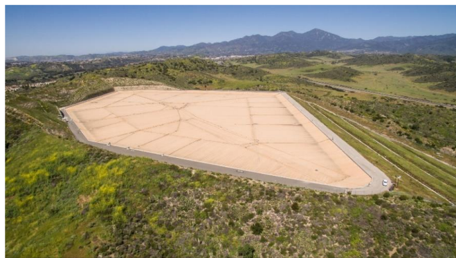
Figure 12. Aerial view of completed Upper Chiquita Reservoir in operations.
